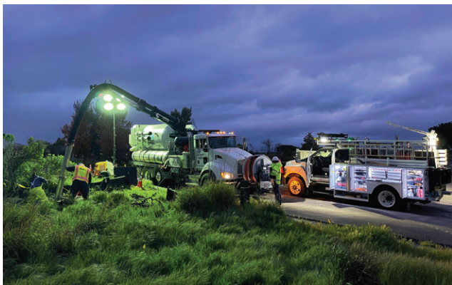
Water Main Repair by City Staff
