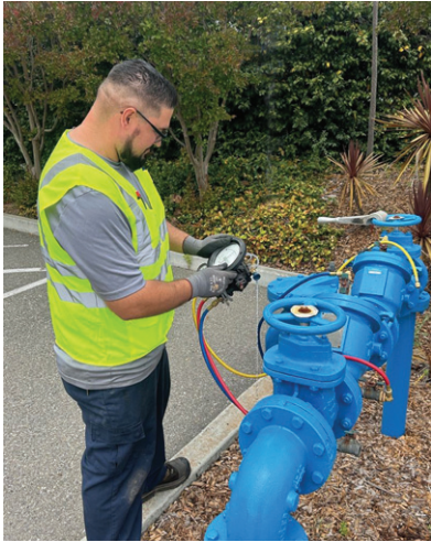
Backflow Device Inspection by City Staff
