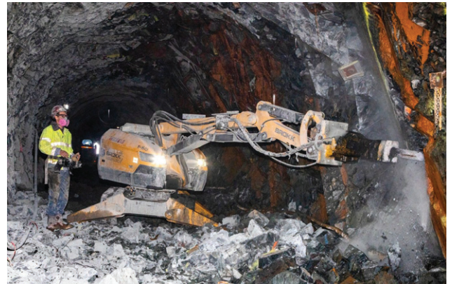
Mountain Tunnel Improvement Project
