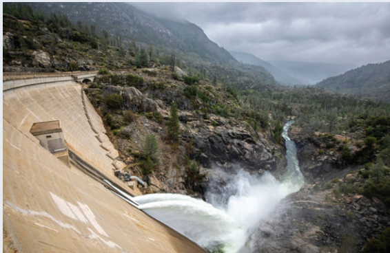
O'Shaughnessy Dam Spillway
