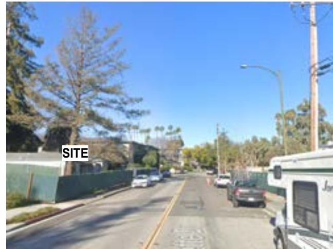
A) EXISTING SITE FROM FAYETTE DR. LOOKING NORTH
