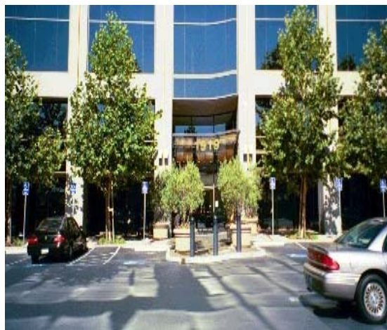
Figure 4-9: Pruneridge Towers, Campbell (Source: Dave Docktor, City of Palo Alto)
