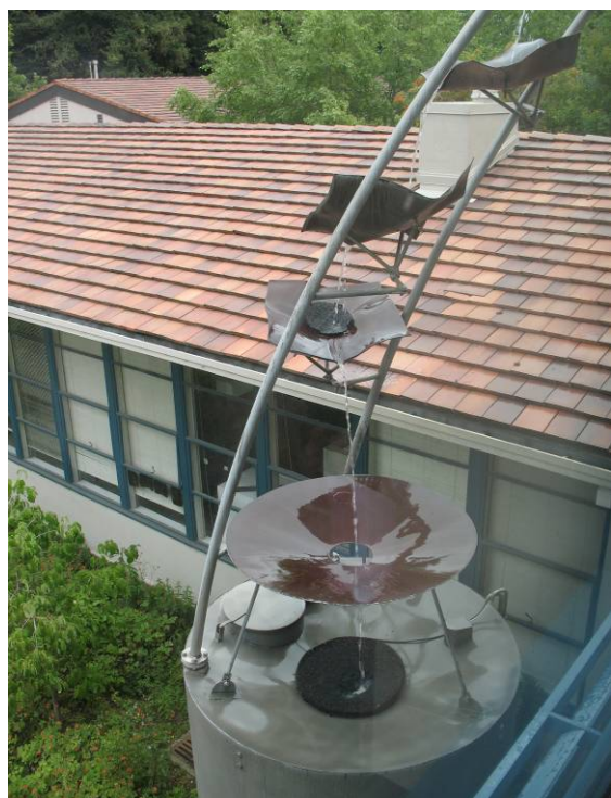
Figure 6-22: Rainwater is collected and used for flushing toilets at Mills College, Oakland.
