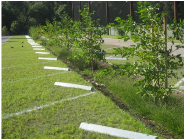
Figure 3-5: Stevens Creek Corridor Park in Cupertino includes turf block pavers in parking lot.
