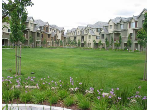
Figure 3-8: This landscaped area in San José also functions as a stormwater treatment area.
