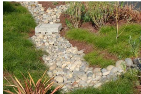
Figure 5-1: Cobbles in this stormwater treatment measure in San José help prevent erosion.
