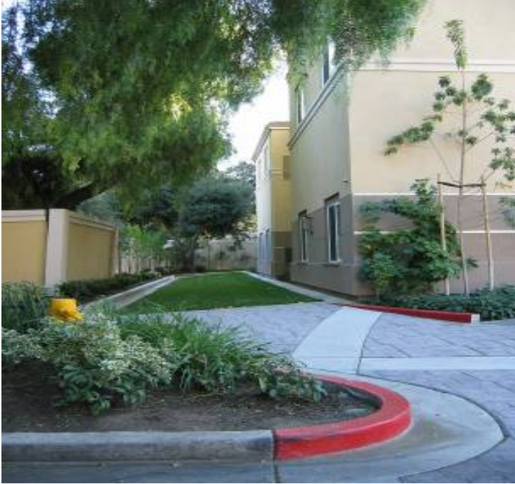
Figure 6-40: Turf block fire access at the Residence Inn in Los Altos
