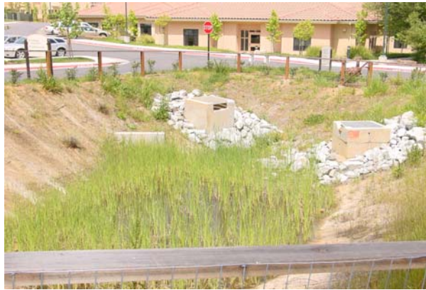
Figure 5-16: Detention pond at a retirement center in Saratoga
