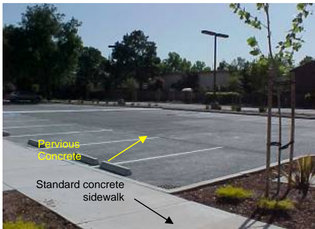
Figure 6-32: Parking Lot with Pervious Concrete, San José
