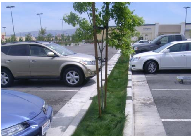
Figure 8-1: Bioretention area at a shopping center in San Jose.
