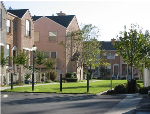
Figure 3-6: A turf block fire lane in Mountain View.
