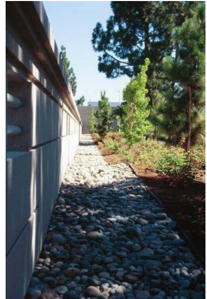
Figure 8-4: Infiltration Trench at former Agilent site, Palo Alto
