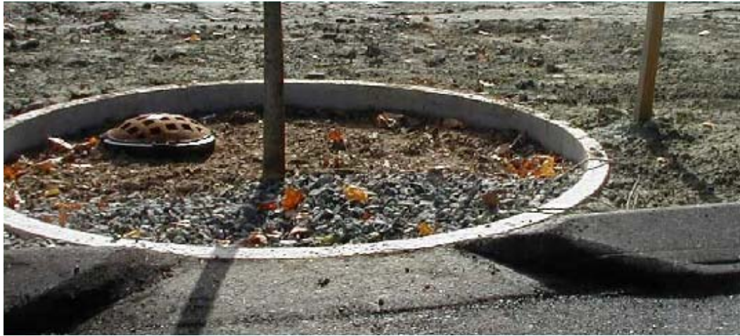
Figure 6-15: Non-proprietary Tree Filter with Overflow Bypass. Source: University of New Hampshire Environmental Research Group, 2006
