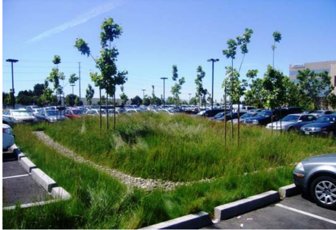
Figure 6-1: Bioretention area in office building parking lot in San José. Source: City of San José.
