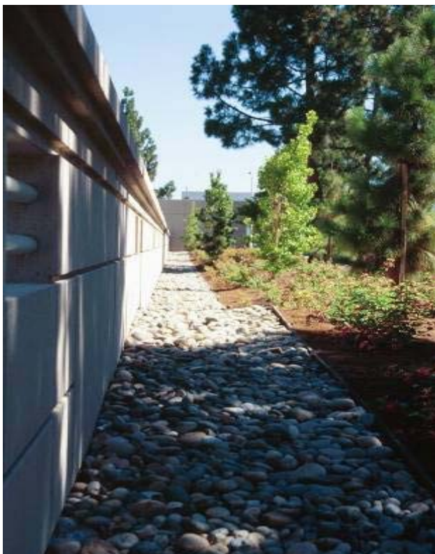
Figure 6-19: Infiltration trench next to parking structure, Palo Alto. Photo: EOA, Inc.
