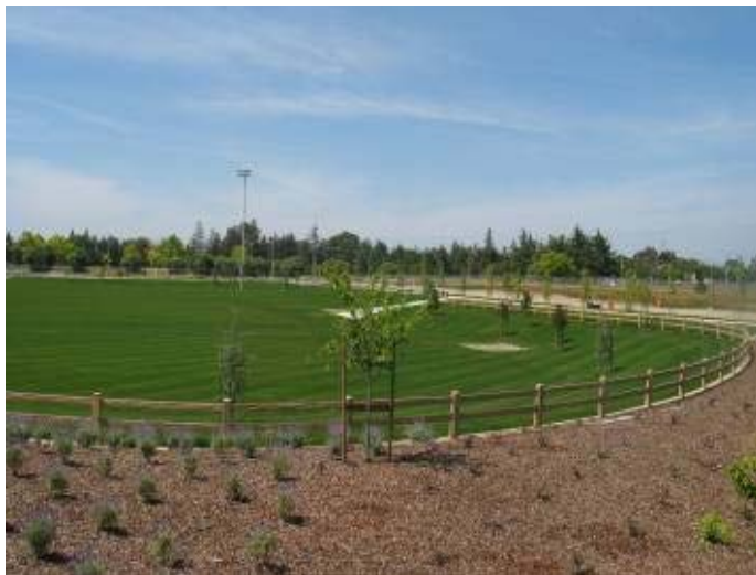
Figure 7-5: Example of a multi-purpose detention facility for HM control in San Jose.
