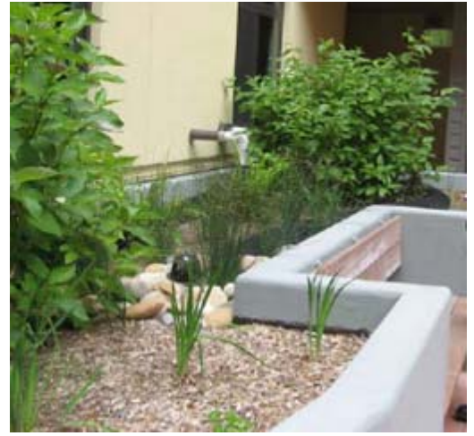
Figure 6-13: The same planter as shown in Figure 6-12, after vegetation has matured and partially conceals the half-buried pipe from view (Source: San Francisco Estuary Partnership).
