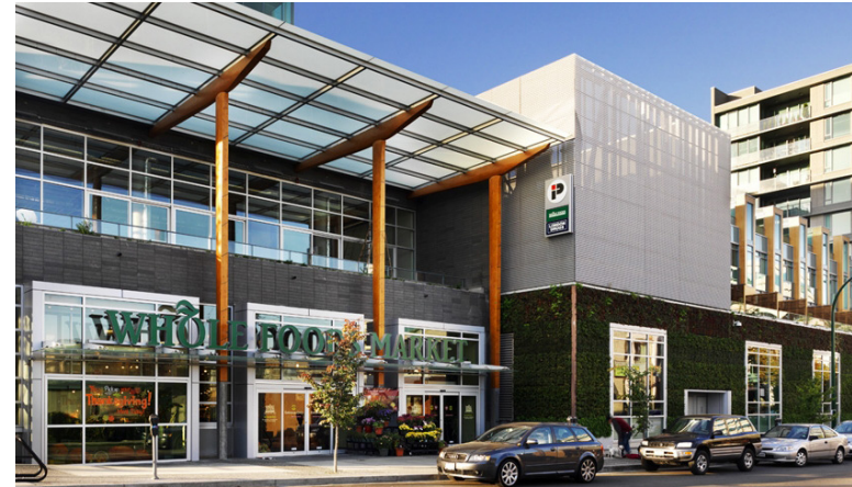
Example of a ground-floor grocery store with high ceiling and windows integrated into a larger mixed-use residential building.
