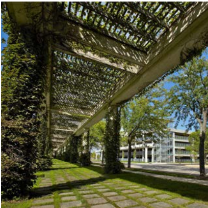
An example of a covered walkway to the parking structure.
