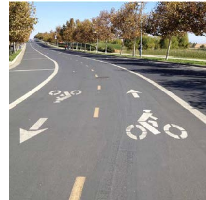
An example of a two-way cycle track next to a bus only lane.
