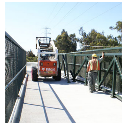
Permanente Creek Bridge construction.
