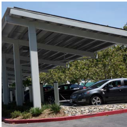
An example of solar shading and electric vehicle charging stations.
