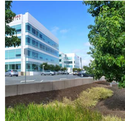
Bioswales adjacent to a surface parking lot.
