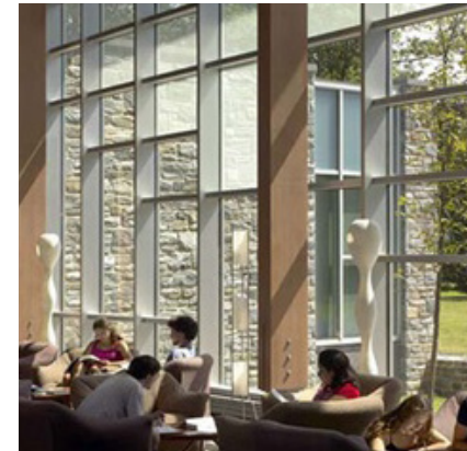
An example of clear glass with bird friendly fritted glass. Rows of closely spaced circles etched in the glass makes the windows more visible to birds.
