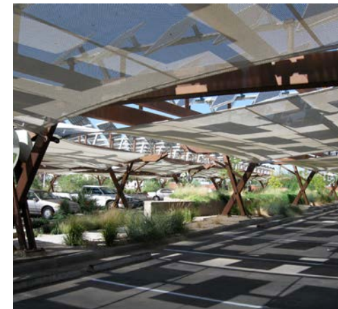
Overhead solar panels provide covered parking and contribute to local sustainability efforts.
