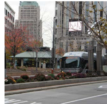
Typical center running transit lane.
