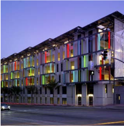
An example of a lined parking structure.
