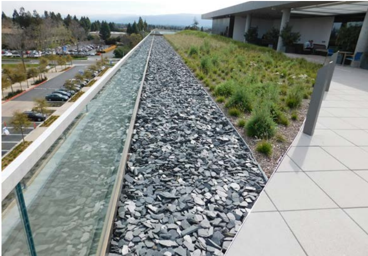
11a. Utilize building technologies and strategies such as solar roofs, green roofs, recycled water and wastewater systems, and transit, bicycle, and pedestrian facilities to help the district become highly sustainable over time.
