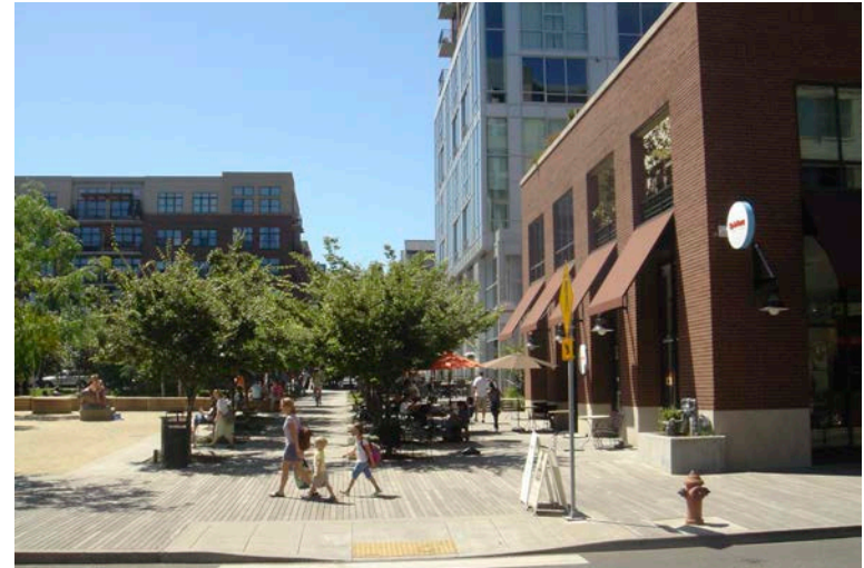
7o. Use visual and physical design cues within a building's design and entries to emphasize pedestrian and bicycle connections to public and natural spaces such as parks, greenways, trails, and open space.
