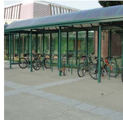
Covered bicycle parking.
