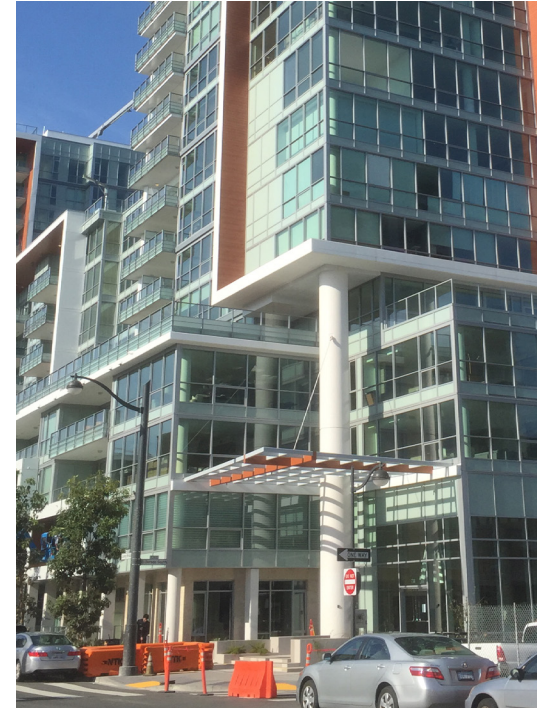
4i. Design upper stories to be slender and graceful in form to reduce their visual appearance of bulk and mass. Upper-story building design strategies may include, but are not limited to, front setbacks, horizontal and/or vertical articulation, building base or podium designs emphasizing human-scale features, and other design strategies. Stepbacks over the building base or podium should balance massing reduction objectives with creating a strong upper-story street presence.
