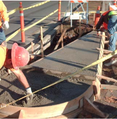
Sidewalk reconstruction in Mountain View.
