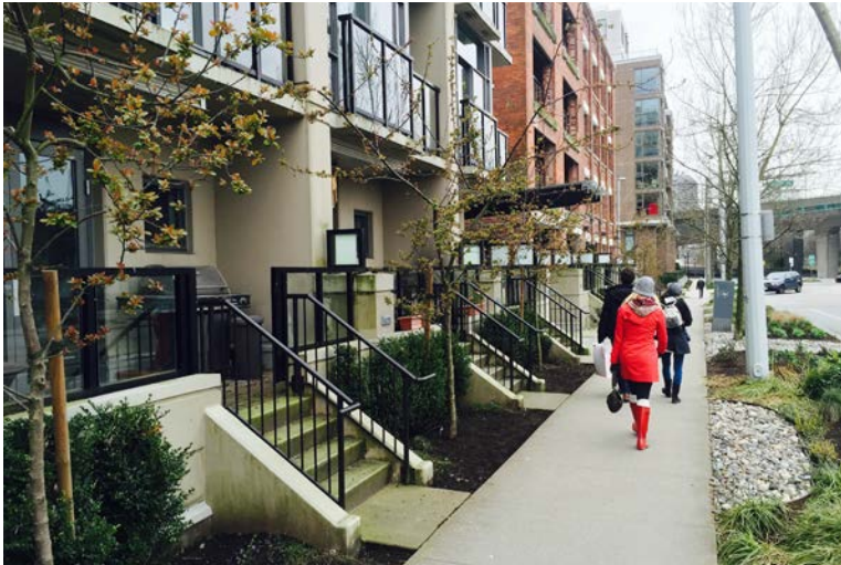
7n. Integrate balconies with a building's massing to generate simple, urban facades. Balconies should employ high-quality materials, design and detailing, including on their underside.
