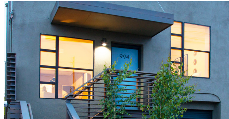
5l. Shelter residential entries from the rain and wind and include an entry light.
