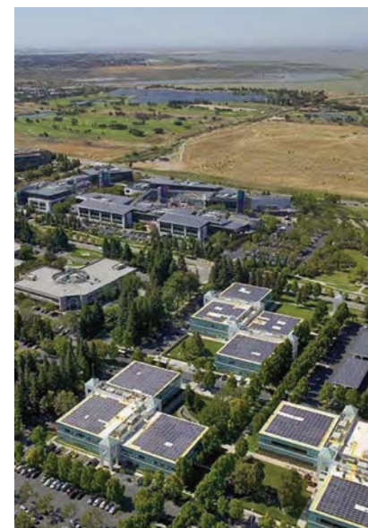
Solar panels on North Bayshore office buildings.
