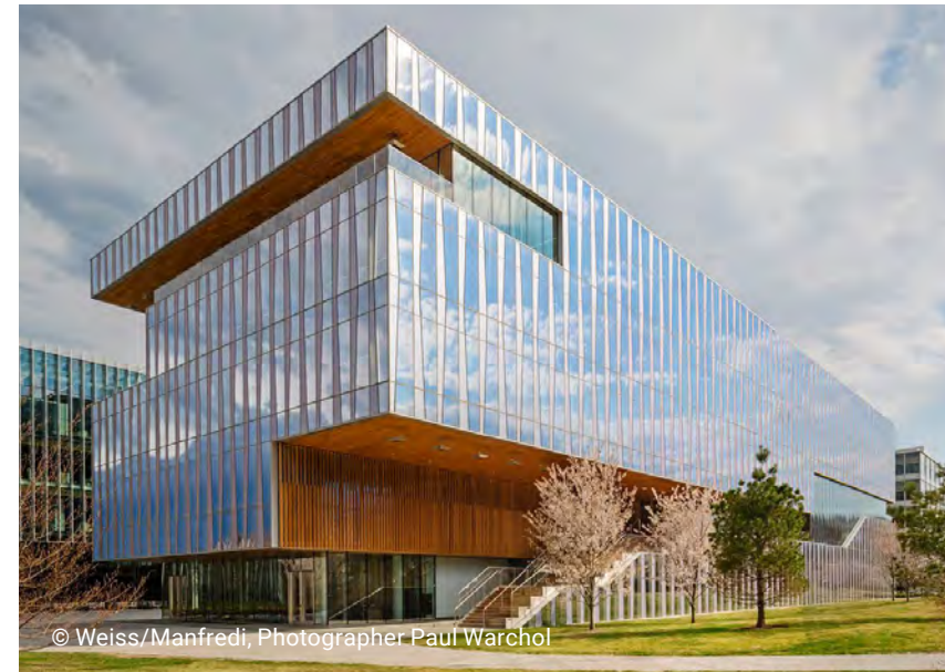
Horizontal massing moves that are visible across the length of the adjacent open space are achieved via setbacks and stepbacks
