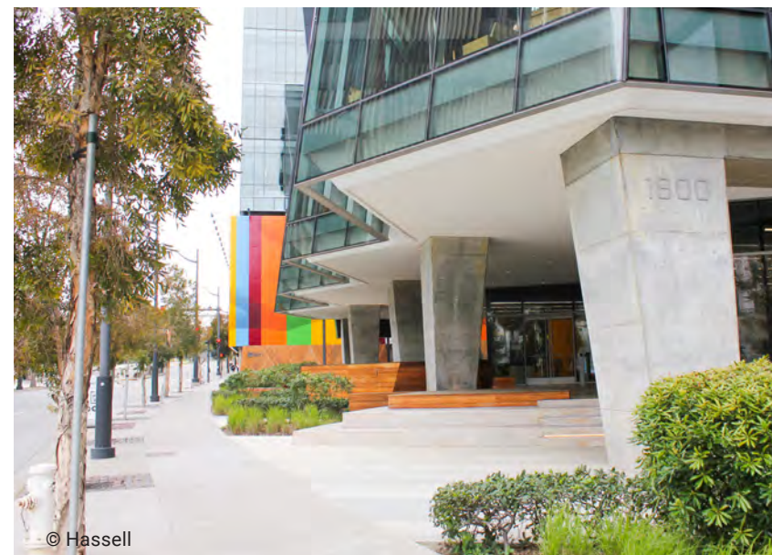
Ground floor setback that creates additional space for pedestrian circulation and seating at the building entry with unique material expressions and/or public art
