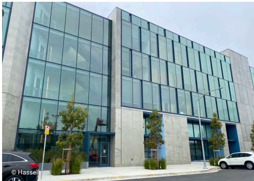
A pattern of recessions help to break the building down into smaller volumes, while subtle shifts in the window articulation add variety to the overall facade
