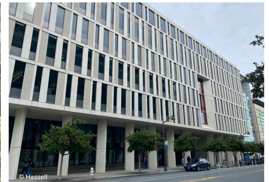
A double-height, recessed ground floor reduces the apparent bulk of the building at street level and creates a shaded/sheltered path of travel for pedestrians
