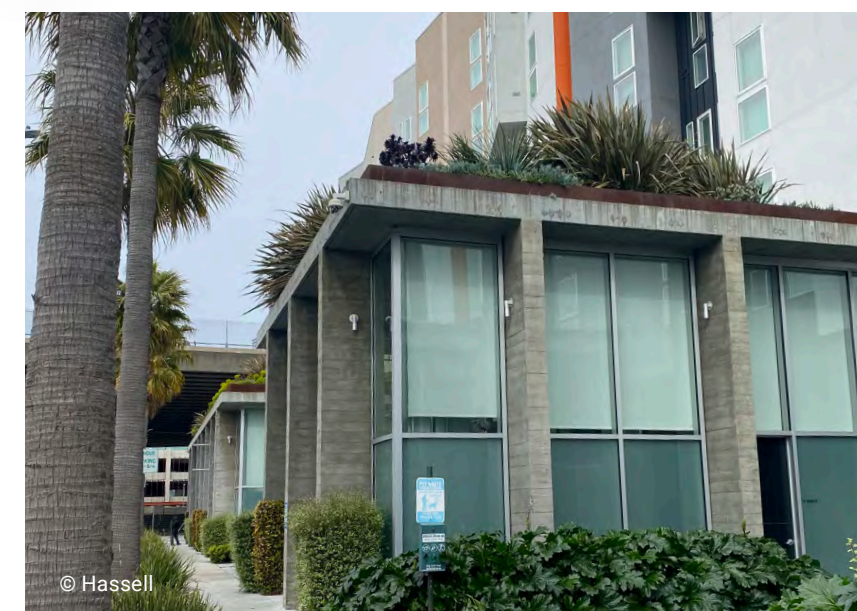
A landscaped stepback above the 2-story base reduces the apparent mass of the building from the pedestrian's view and increases the diversity of the streetscape
