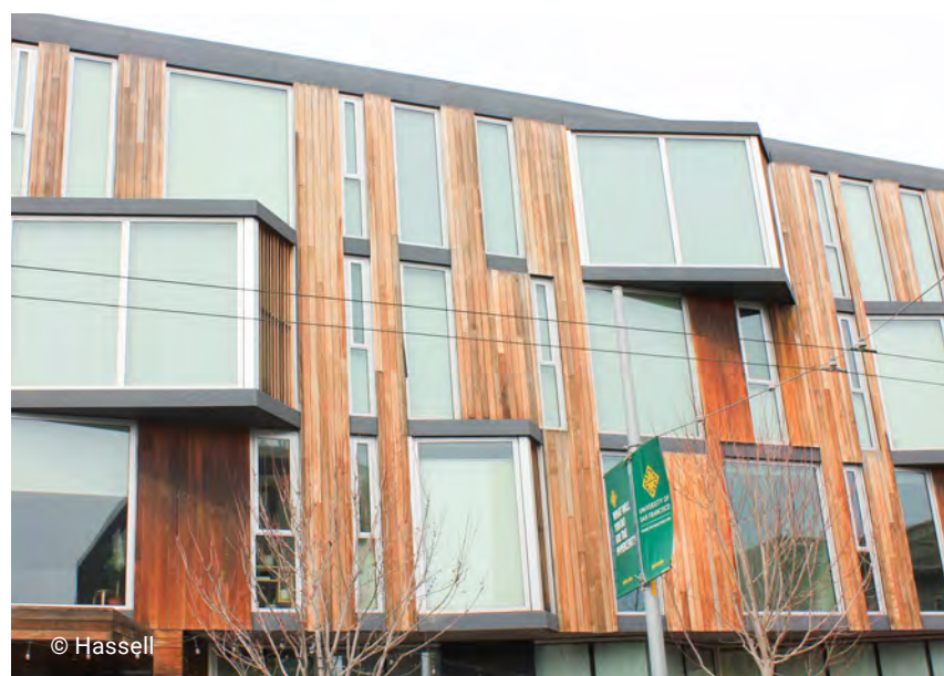
Minor massing expressions in the form of projected bays along the length of the facade articulate individual rooms
