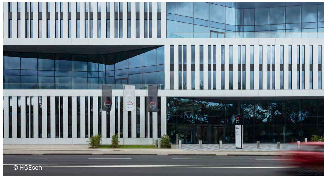
Longer horizontal building expressions achieved using setbacks and stepbacks that are visually engaging at both pedestrian and vehicle speeds of travel
