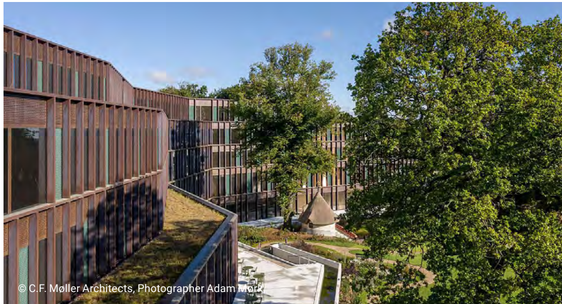
A planted stepback above the building base serves as a large scale horizontal massing move along the adjacent open space and contributes to the natural surroundings
