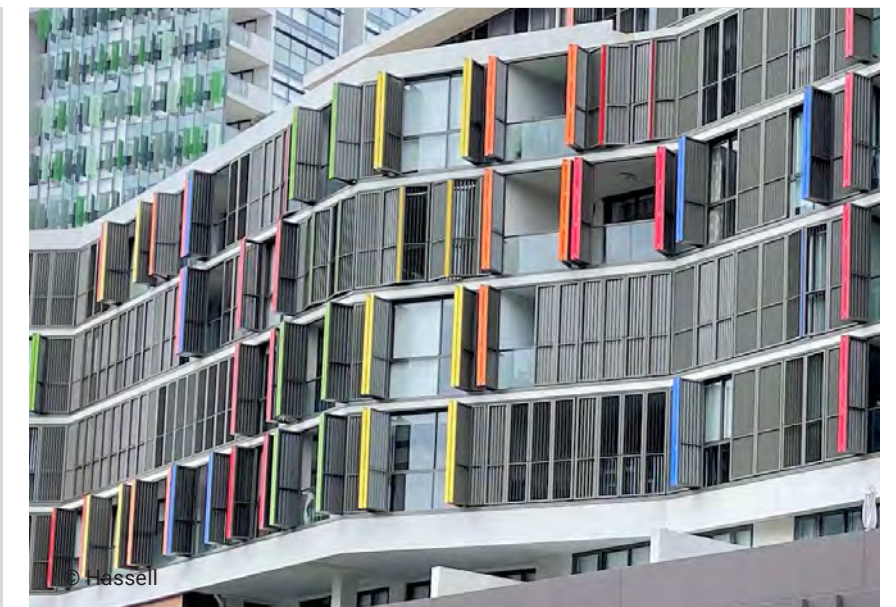
Consistent changes in facade depth and material help reinforce the breakdown of the overall building mass across the length of the facade
