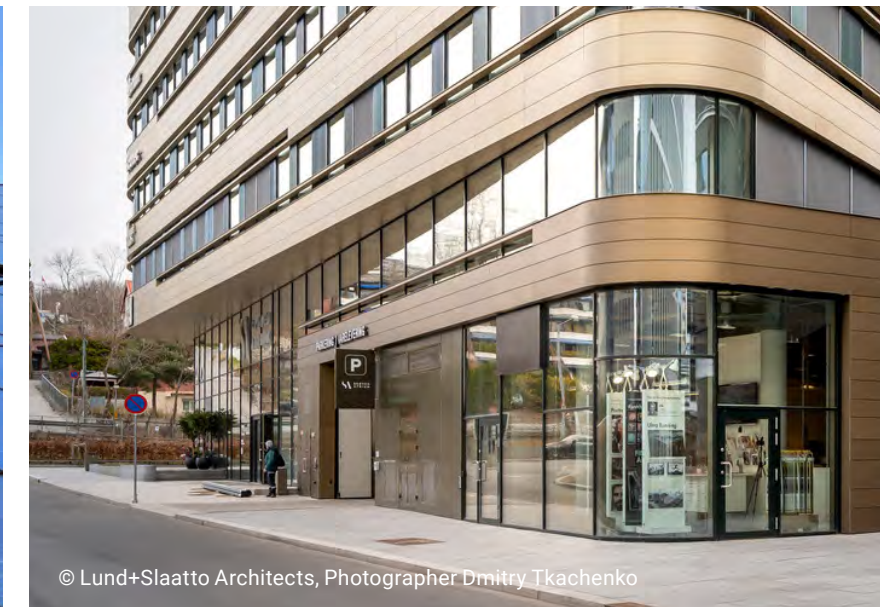
A recessed ground floor provides a clear massing move that engages the street and creates definition from the building above
