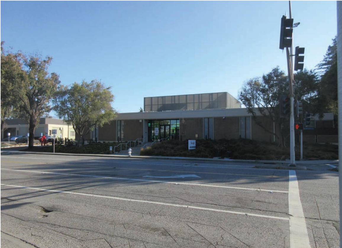
Photo 1: View from the northeast corner of the San Antonio Road and Bayshore Parkway intersection looking east towards the project site.
