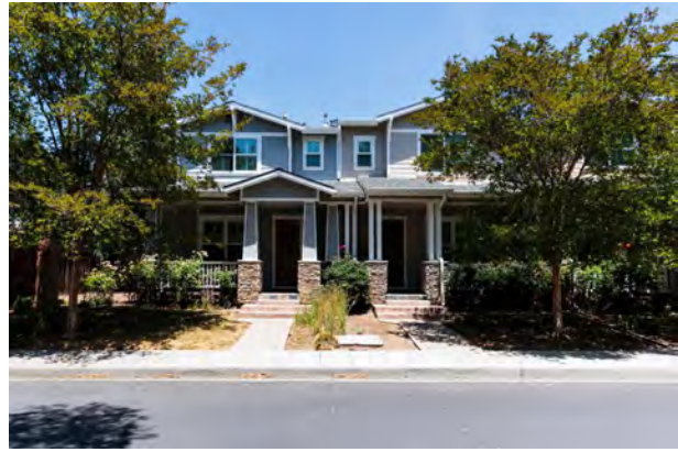
A rowhouse development on Willowgate Street
