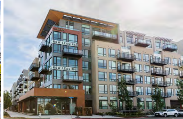
Example of a precedent project in the San Antonio Precise Plan – 400 San Antonio Road
