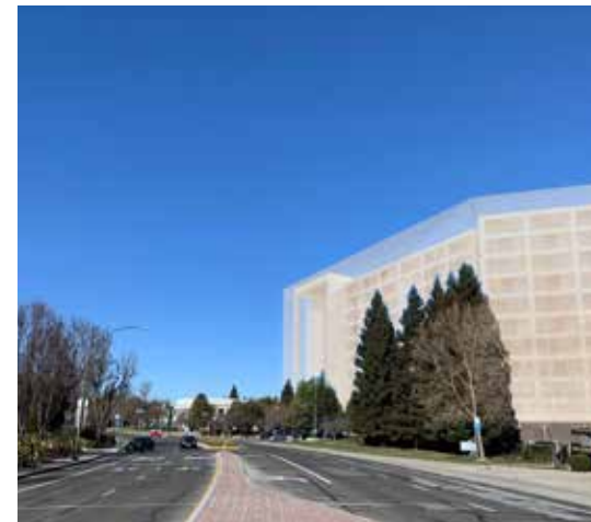
Ellis Street and Middlefield Road looking west near VTA tracks
