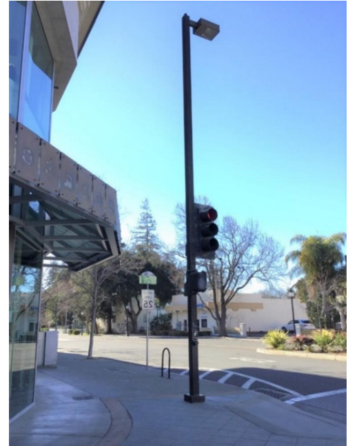
Figure 13 - Existing Shoebox Style Flood Light
