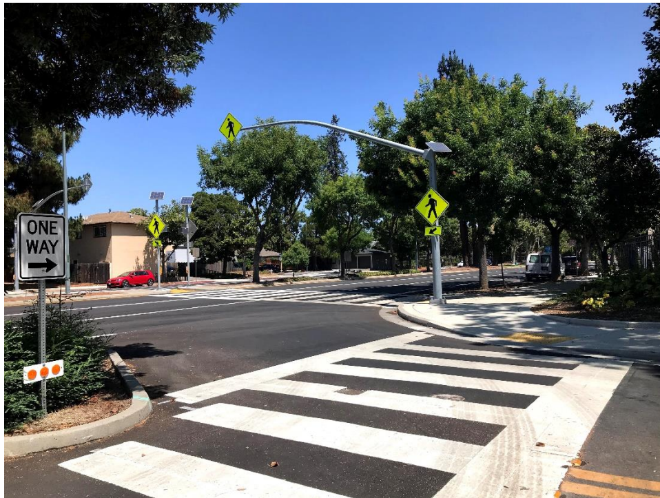
Figure 3: LED-Enhanced Pedestrian-Activated Flashers across Shoreline Boulevard
