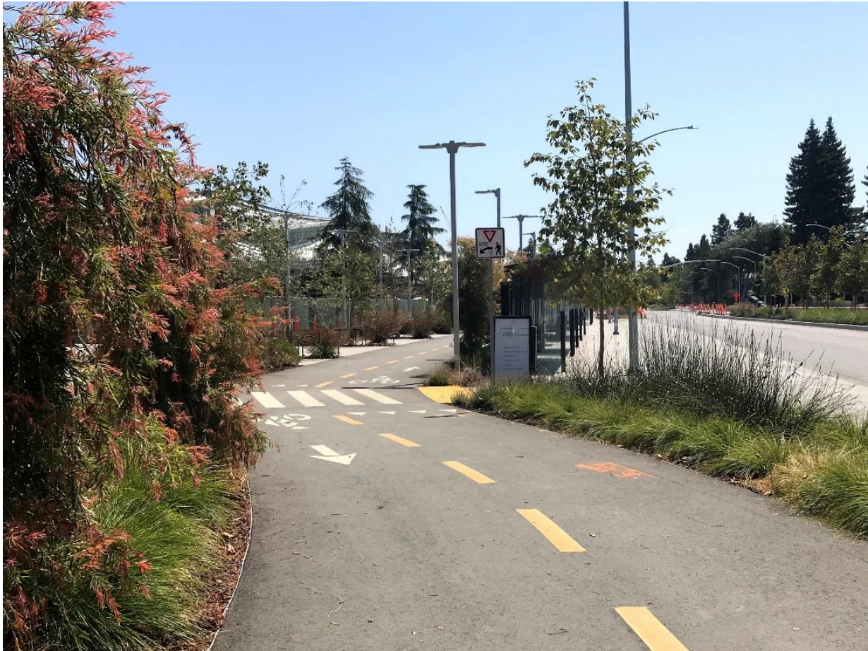
Figure 8: Two-Way Class IV Cycle Track with Development on Charleston Road
