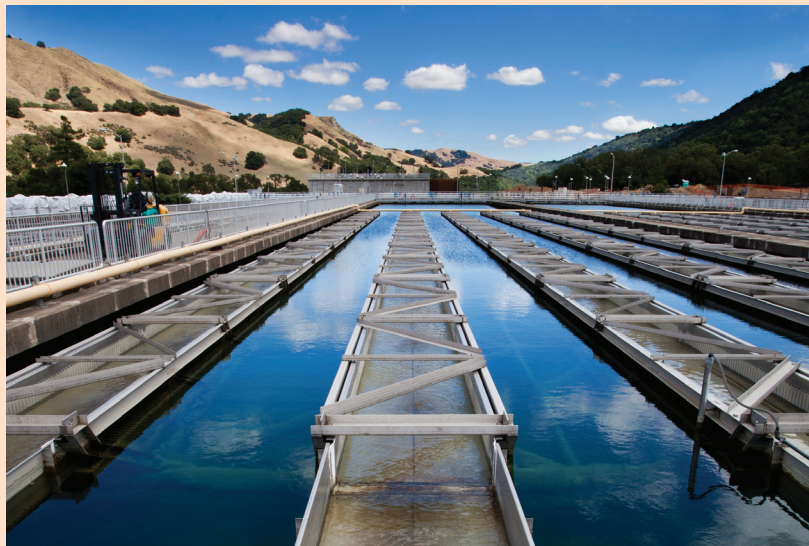
Sunol Valley Water Treatment Plant
