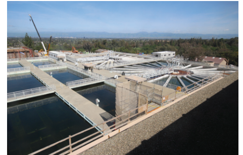
Rinconada Treatment Plant photo: SCVWD
