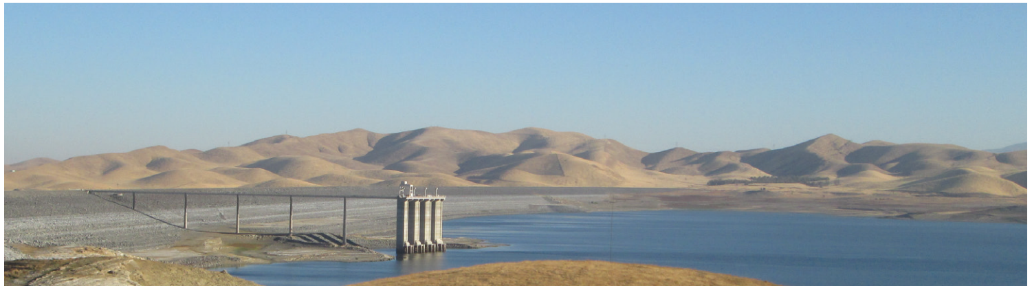
San Luis Reservoir, October 2015
