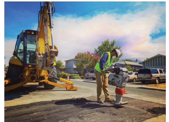
Water main repair by Mountain View staff photo: Gary Wheaton
