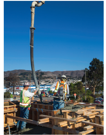
SFPUC Groundwater Storage and Recovery site construction
